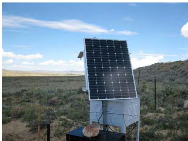
System with large external battery box (July 2011)
