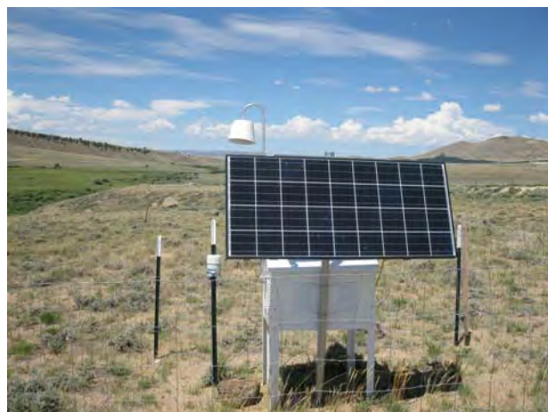
System with battery box inside Enclosure (July 2011)
